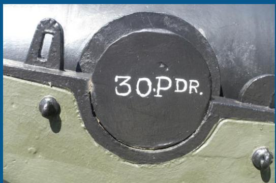
The face of the left trunnion confirms the weight of the projectile
